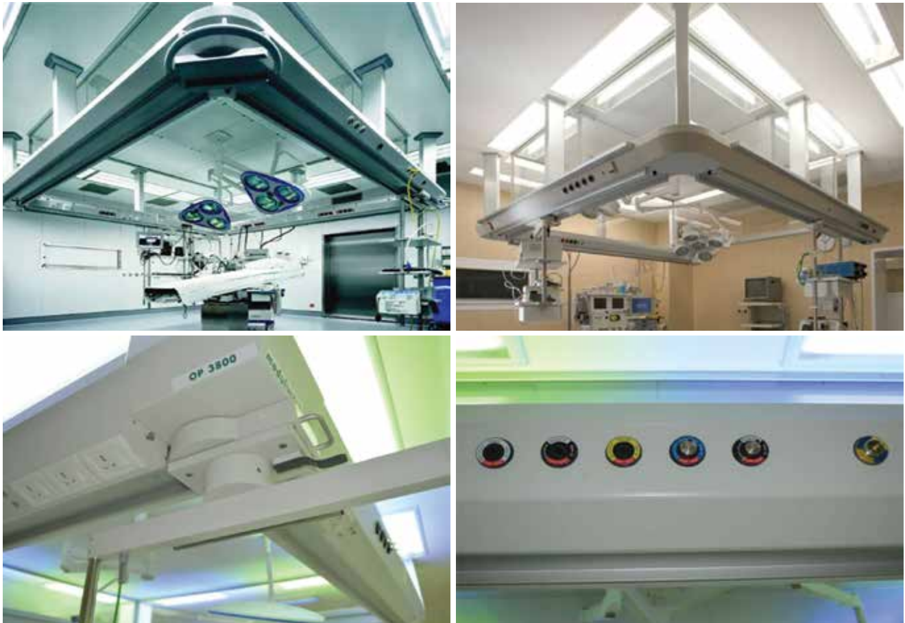
Fig. 4: Media bridge of an integrated OT (showing its various components)
